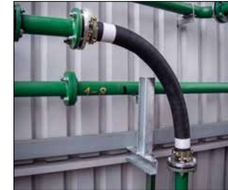
● Kalflex used as flexible pipe bend
