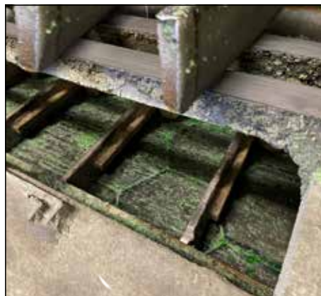
● ABRESIST glass cullet conveyor
